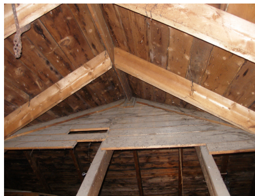
Evidence that both roofs has been built at the same time. No trace of shingle nails.
